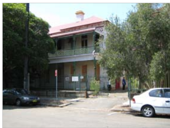
Picture 6 – Chief Mechanical Engineers Office Building
