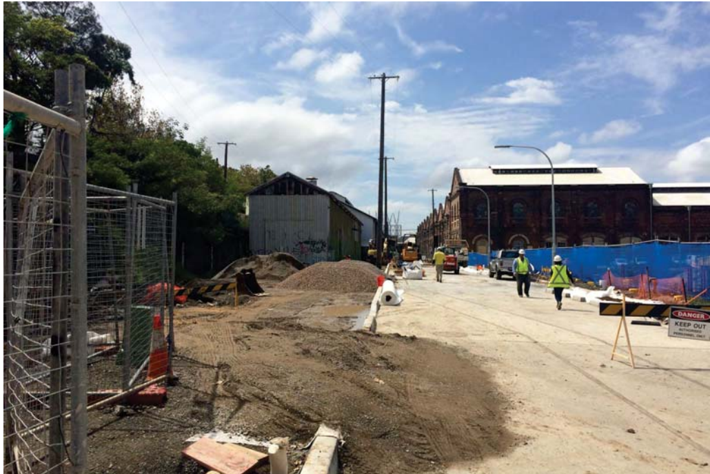
| Construction of Carriageworks Way, North Eveleigh
