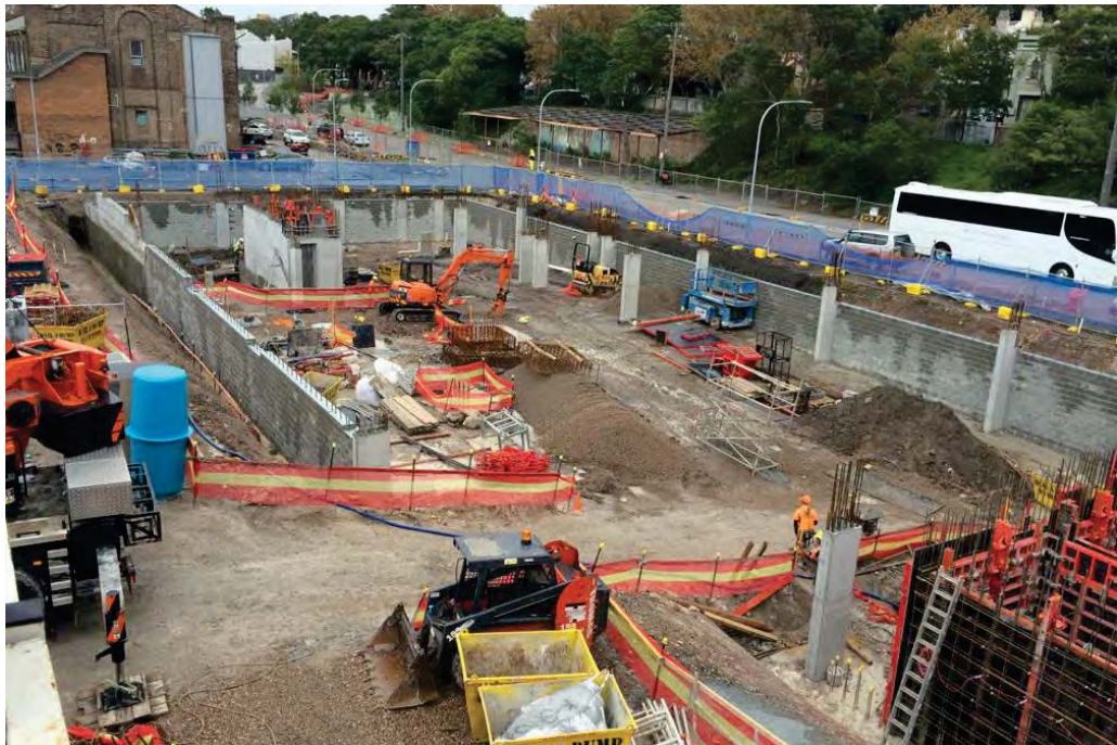
| Construction of Platform Apartments, North Eveleigh
